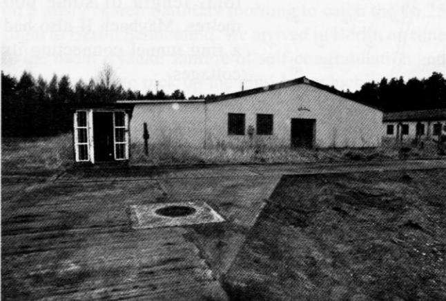
The surface building above the entrance to 7007
